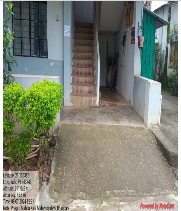
STAIRCASE AND RAMP OF THE BUILDING
